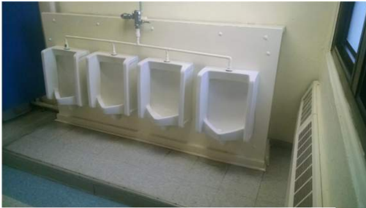
EXISTING BOYS TOILET ROOM
